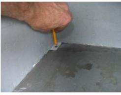
2. Place the unit on the flat base and mark the holes in the stainless steel mailbox feet. Add cross hair marks as a drilling reference.
