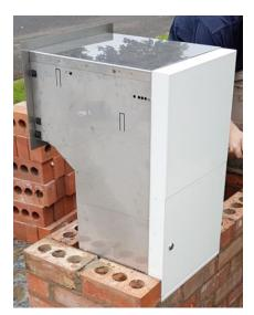
Plumb the parcelbox, packing under the feet if required.
