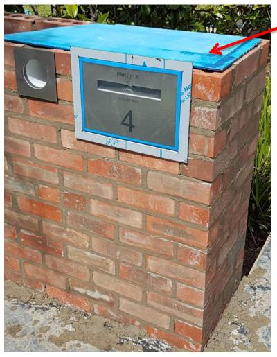
Waterproof cement sheet or lintel approx. 8mm thick. If it is bowed, locate the bow upwards. You must prevent the letterbox roof sagging down, esp. at the front, as this could jam the front door.
