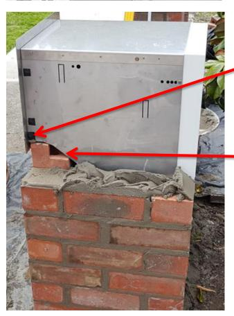
Cut the bricks at the front to clear these weld nuts. Up to 20mm gap is OK at the front, because the door surround covers 30mm all around the front door.
