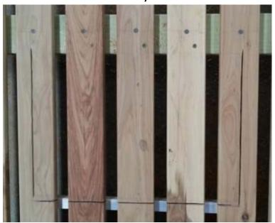
5. Cut the top end of the pickets 4-5mm above the underside of the rail to allow water to drain to the sides. Also add large drains under the top rail at either side as shown, angled downwards.
