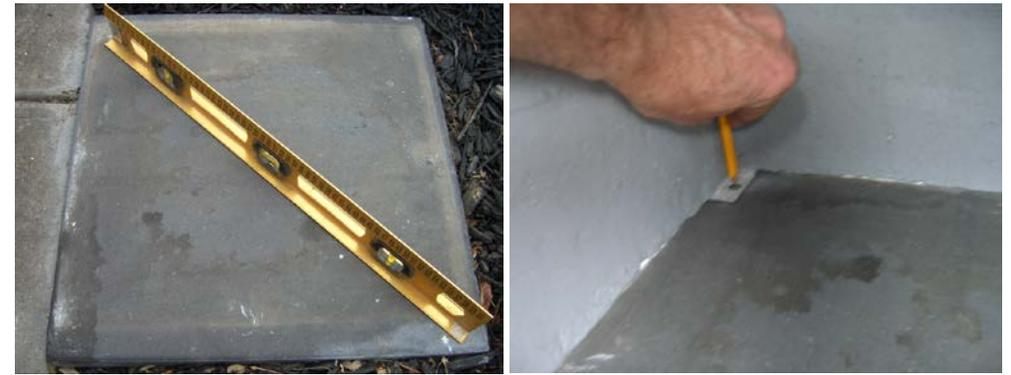
2. Place the unit on the flat base and mark the holes in the stainless steel mailbox feet. Add cross hair marks as a drilling reference.
