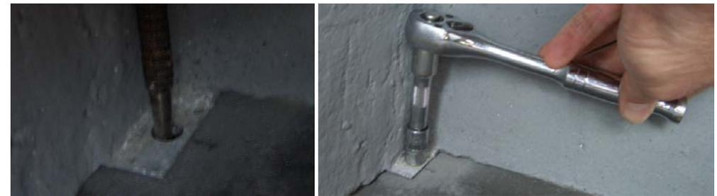
6. Insert the Dynabolts in the holes and tighten. Do not overtighten, as this could break the feet free of their embedments in the letterbox shell.
