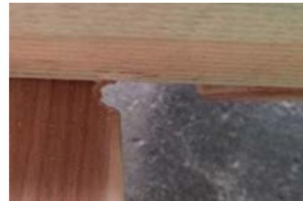
6. Cut recesses for the door pivot weld nuts (lumps on outside).
