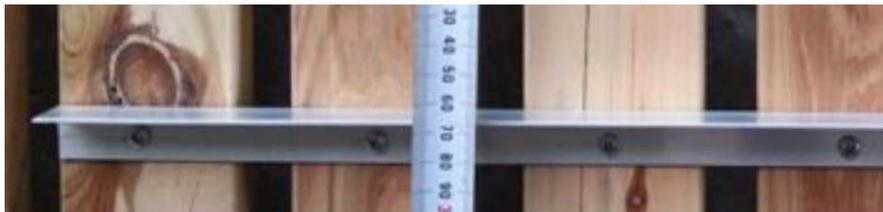
3. Predrill and add extra screws at the top rail so the pickets do not rotate.
